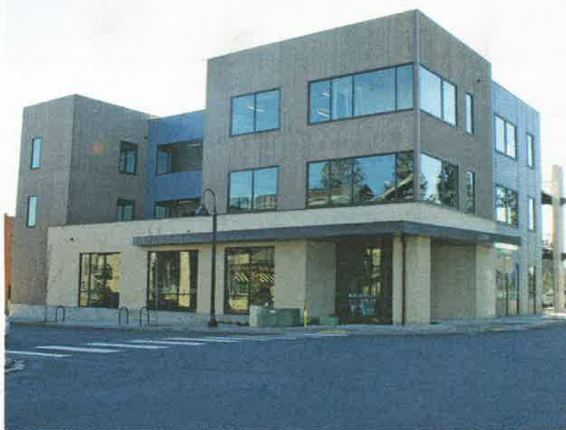
THE CLEARWATER CROSSING BUILDING | PHOTO BY RONNI WILDE
